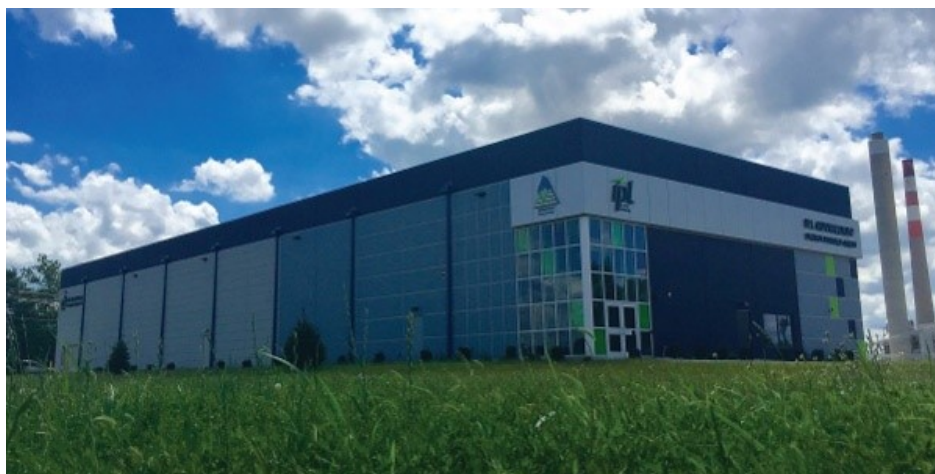
Indianapolis Power & Light's Harding Street Station storage facility | U.S. Department of Energy
